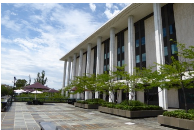
Figure 9. Patterned paving on Podium
