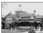
Grant Ellmers Brick and Marseille Tile Edwardian House, Webster Street, Ballarat, Victoria 1994
